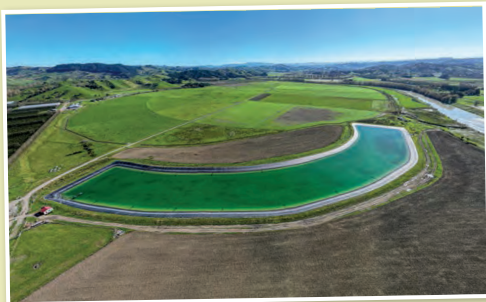
250,000 cubic meter water storage pond on Tangihanga Finishing Farm. Dimensions are 700 meters long, 100 meters wide, 5 meters deep and a surface area of 4.5 hectares.
